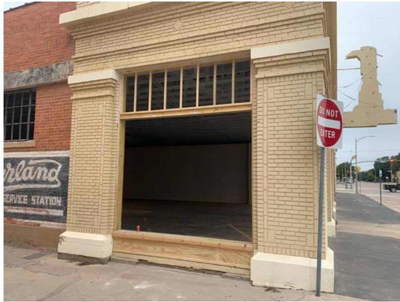
Figure 4: 1149 N. 2 nd alley Store Front Window Casing
