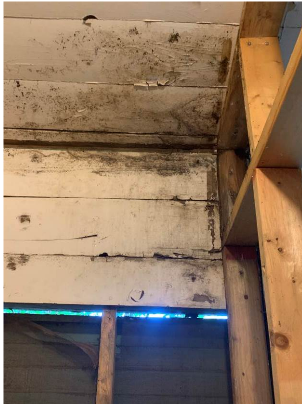
Figure 7: Porch interior view of damaged wood siding
