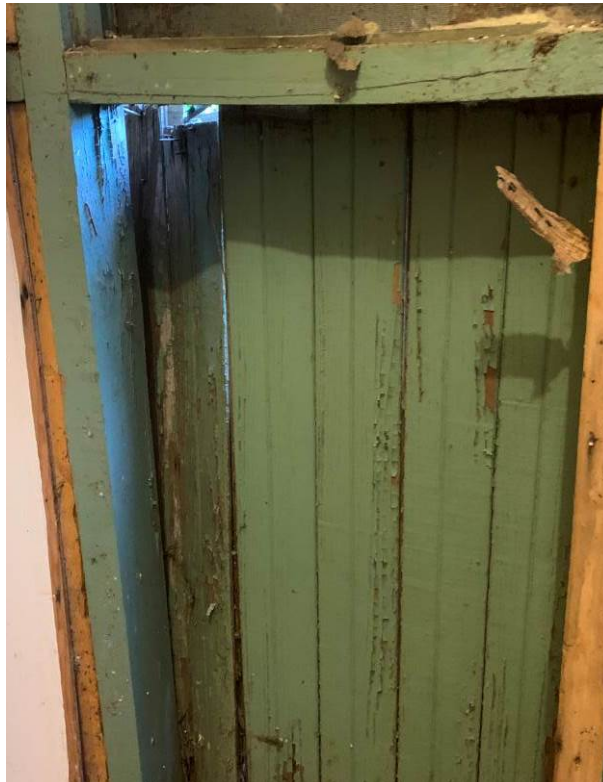
Figure 7: Porch interior view of damaged wood siding
