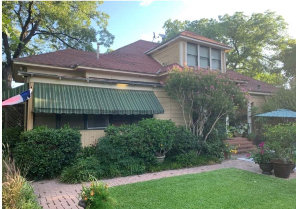
View of South facing Porch
