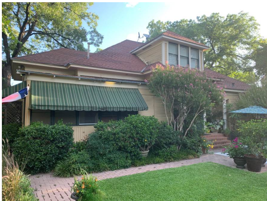
Figure 1: View of Damaged Porch
