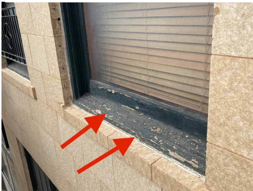
Figure 4: Deteriorated paint at center of exterior window
