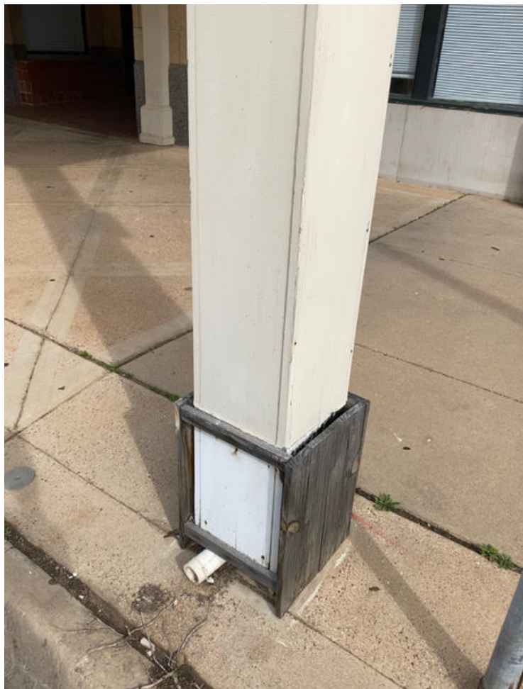
Figure 8: Unfinished column at store front
