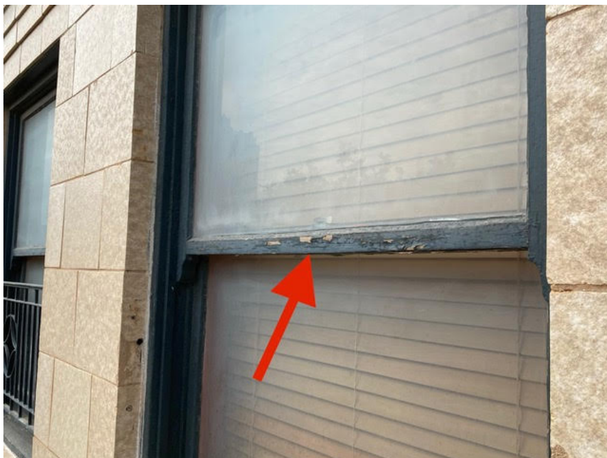
Figure 4: Deteriorated paint at center of exterior window
