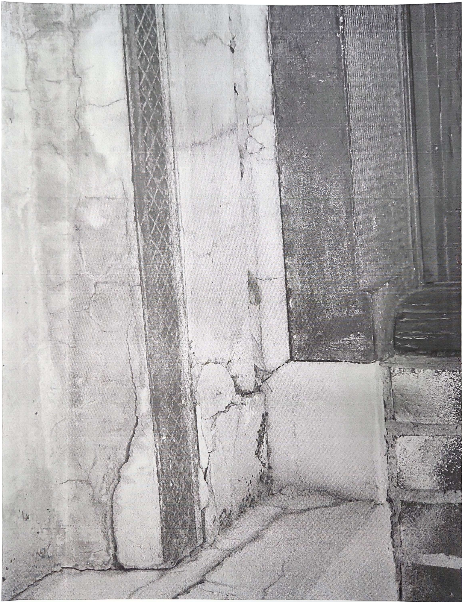
West side of Building - Entrance way
