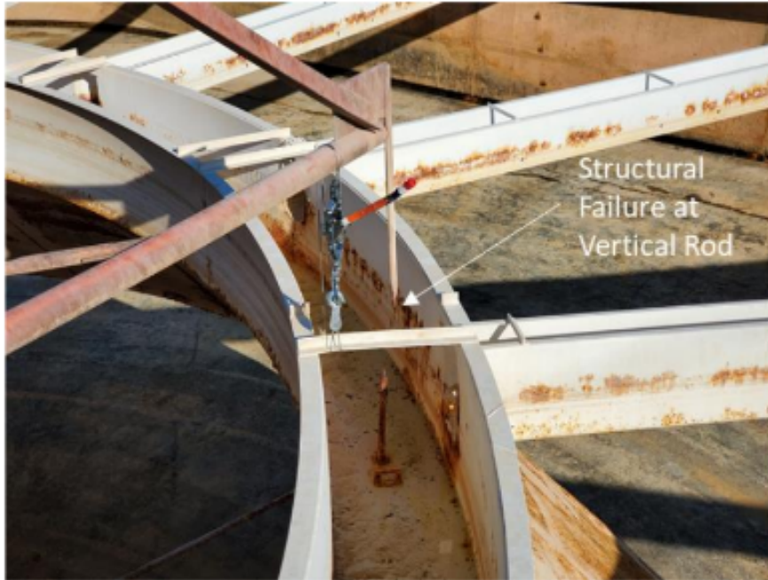
Figure A.1 – Clarifier Structural Failure Site Photos
