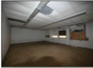
SECOND FLOOR PHOTO 2
