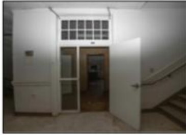
SECOND FLOOR PHOTO 4
