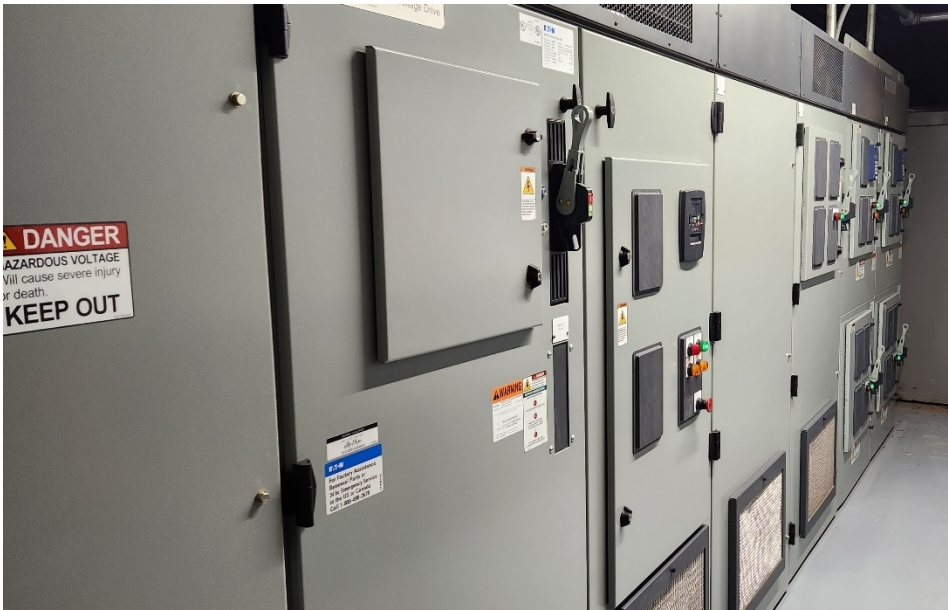
New Variable Frequency Drive Units
