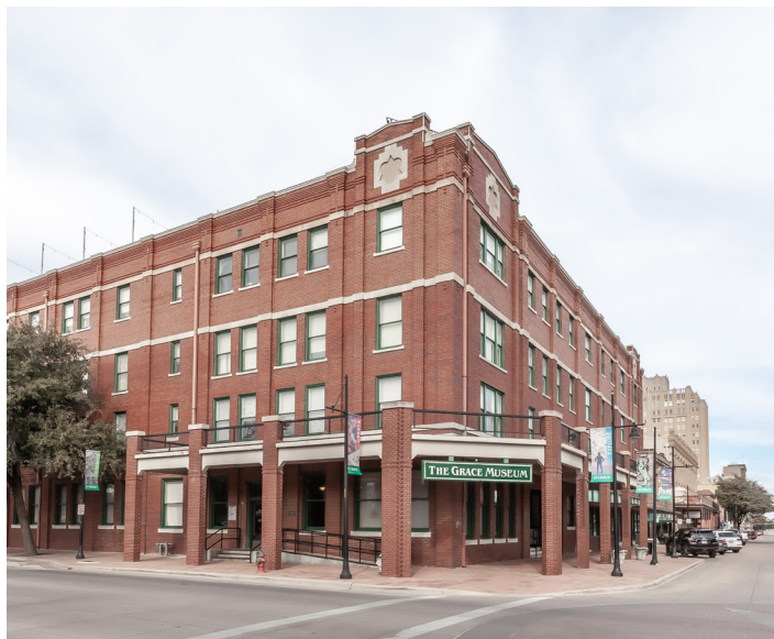
The Grace Museum was one of the first historic structures to be renovated in Downtown Abilene. It's success launched the revitalization of Downtown.
