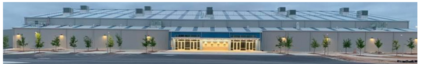
The renovations and expansion at the Taylor County Expo Center already are attracting new business.
