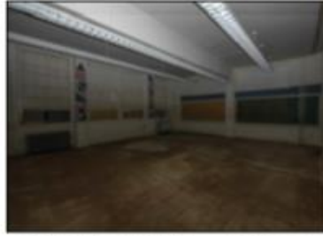
SECOND FLOOR PHOTO 6
