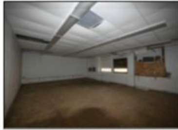
SECOND FLOOR PHOTO 2
