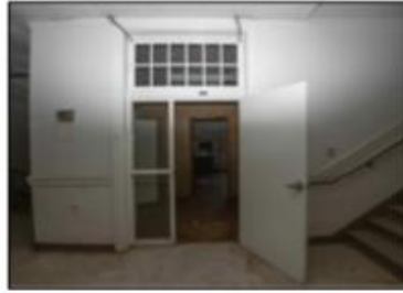
SECOND FLOOR PHOTO 4
