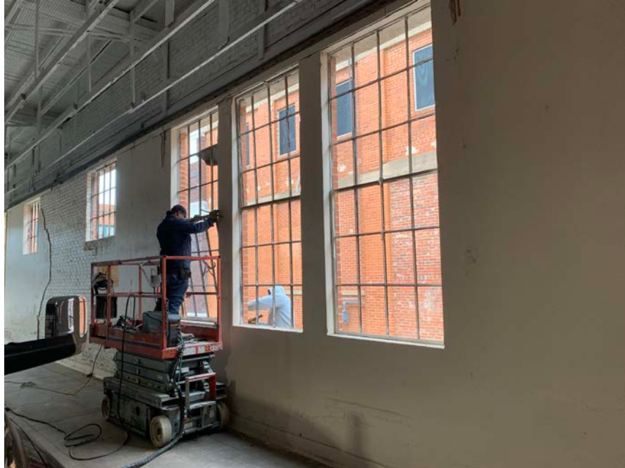
Figure 5: Steel Window Casings
