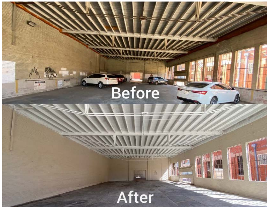
Figure 12: 151 Cedar St: Before and after photos
